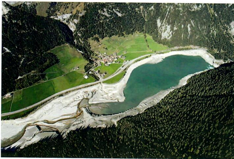
Sediment depositions in Sufers Reservoir, Switzerland, during drawdown (Courtesy Kraftwerke Hinterrhein)
