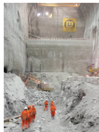
Figure 4 | Excavation of main machine hall of the underground powerhouse of Limmern pumped storage powerplant in Switzerland. [Courtesy Anton J. Schleiss].
