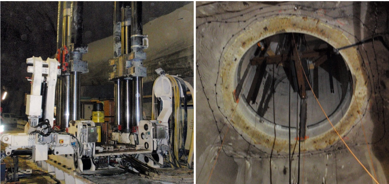
Figure 2 | Left: Raise-boring equipment at the top of the vertical pressure shaft of Nant de Drance pumped storage powerplant in Switzerland. Right: View into the concrete lined vertical pressure shaft from the bottom. [Courtesy Anton J. Schleiss].
