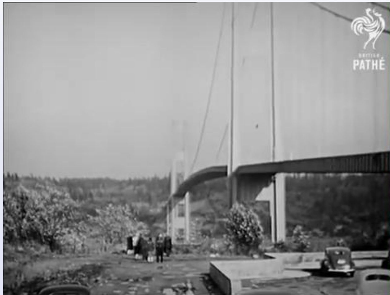
Collapse of the Tacoma bridge
