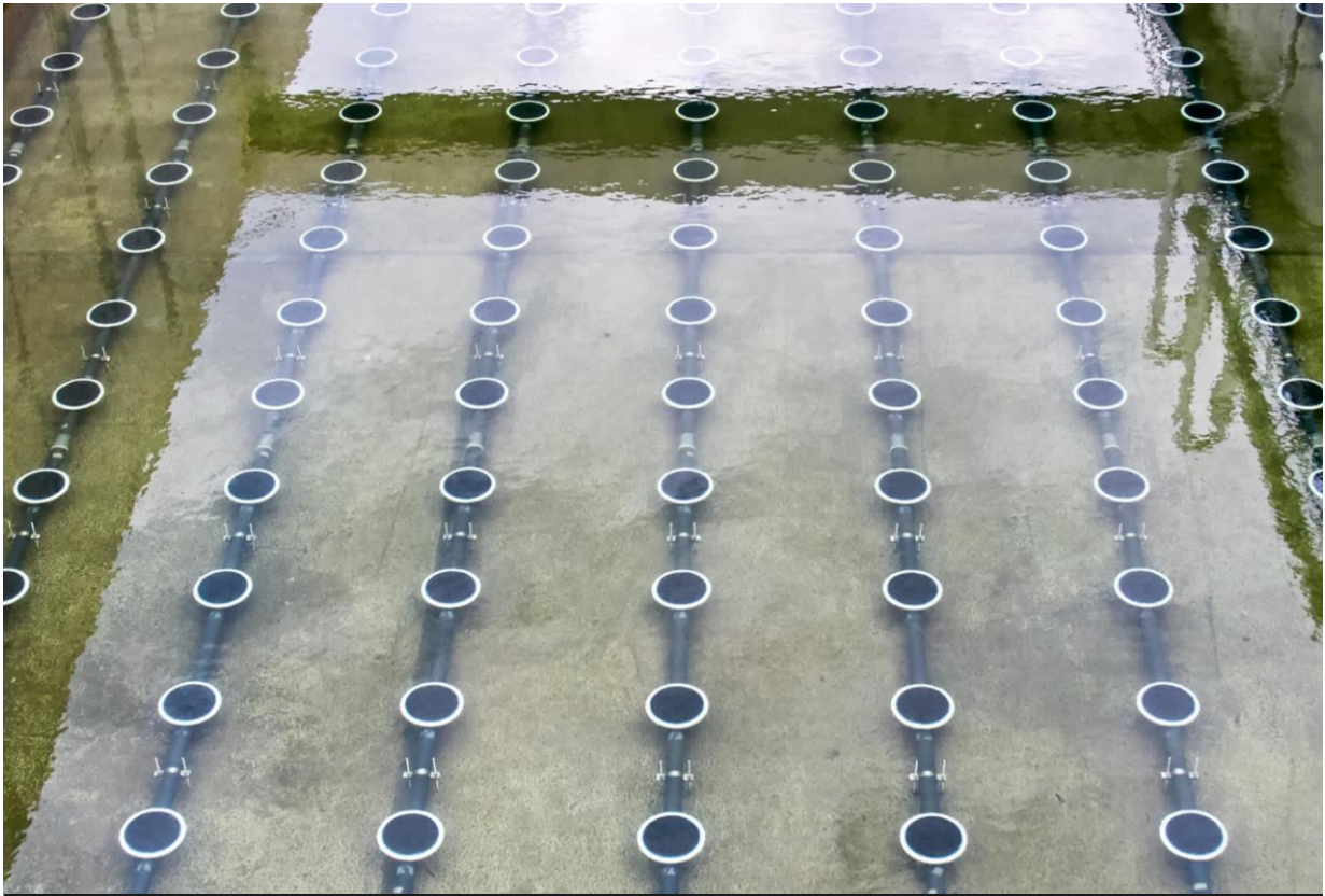
Membrane Diffuser
