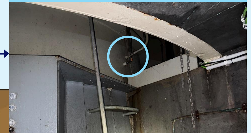
Draft Tube Cone Pressure Sensor
