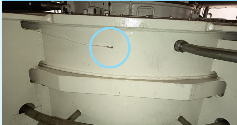
Generator Accelerometers
