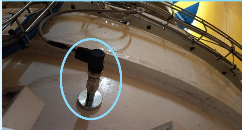
Head Cover Accelerometers
